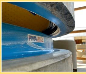
FULLY LINED MANHOLE INCLUDING JOINT LINING
