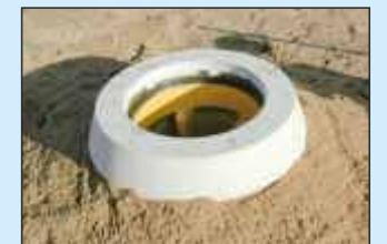
The concrete load distribution ring disconnects the heavy loads
