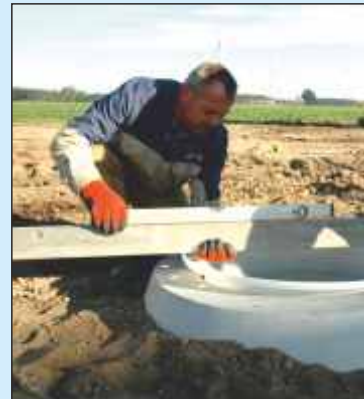
The adjustable telescope can be aligned to the road level
